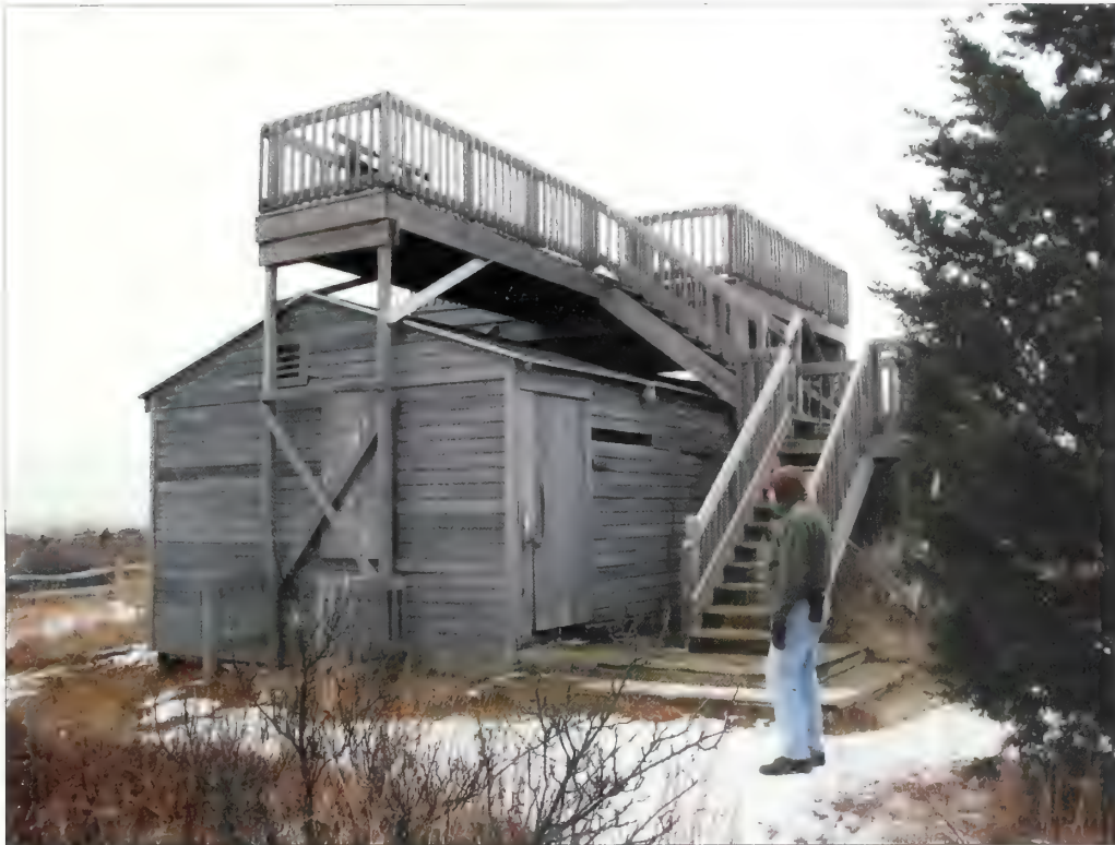
Figure 3.13. View looking northeast at observation platform. North of Batteries Engle and Peck, an observation platform stands on top of a one story, wood-frame structure. The platform permits panoramic views across Lower New York Harbor and is regularly used for bird watching (Olmsted Center, January 2009).
